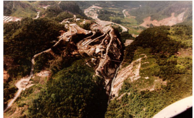
View From Up-Stream
